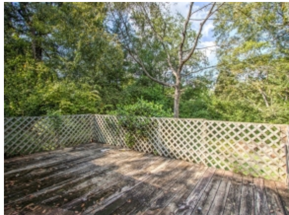
Wood Deck to Backyard
